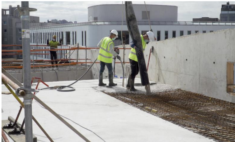
Coulages dalles – Piscine Pantin (93)
