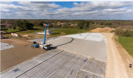
Dalle de stockage Argilus, 3 000m 2
